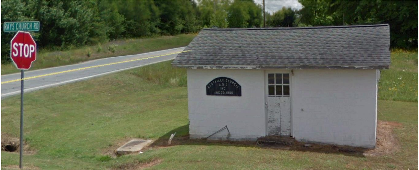
Building in Southeast quadrant.
