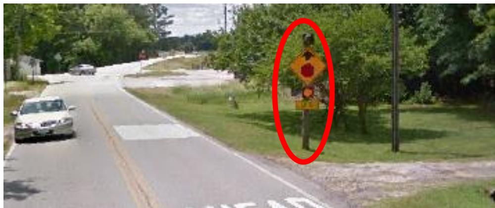
Figure 7. Single Indicated STOP Ahead Warning Sign With Flashing Beacons
